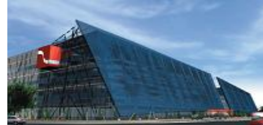
1MW on-grid BIPV System for Suntech's new R&D Center in Wuxi, China
